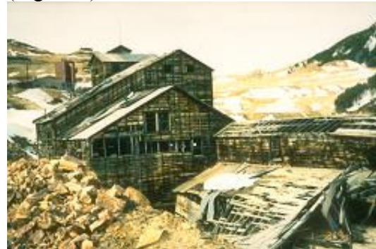
Figure 2. Historic Ruby Mill with active cyanide heap leach pads in upper right background.
